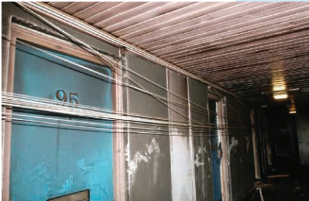
Post incident photograph of the eleventh floor landing showing displaced cables.
