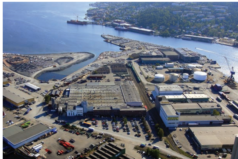
Inter-array connections facility in Drammen, Norway, manufactures submarine cables for offshore wind farms
